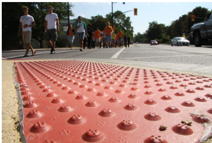
Photo of new detectable warning surface at road crossing. Courtesy of Paul Mayne, Western News
