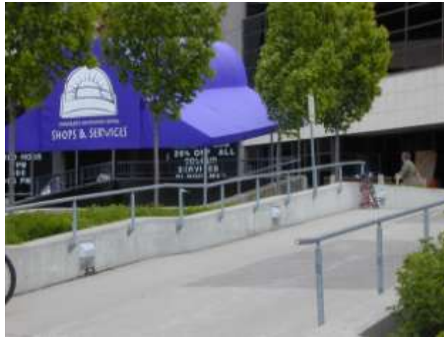
Accessible ramp at the University Community Centre
