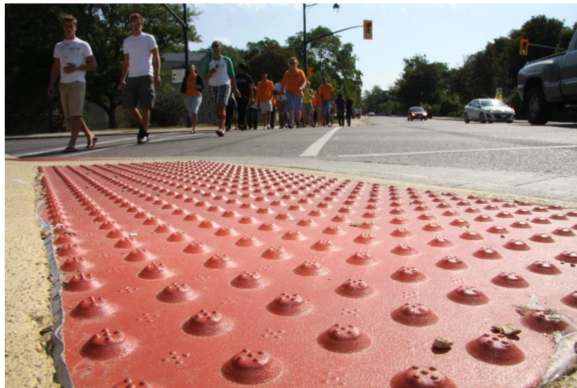
Photo of detectable warning surface at road crossing. Courtesy of Paul Mayne, Western News
